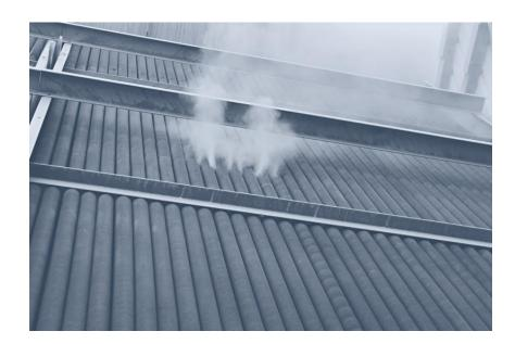
Within the framework of a routine maintenance programme and with the aim of restoring an appropriate heat exchange for this kind of equipment, CTP environnement suggested cleaning the finned tubes using its Decamex® process.
